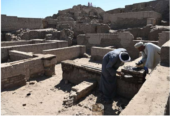
Fig. 5: Consolidation of mud-brick wall in House BC (photo: O. Kassab, © DAI).
